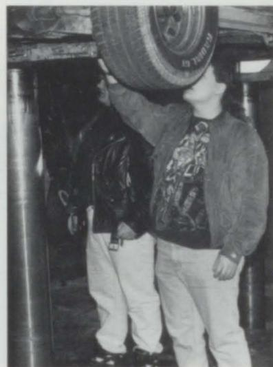
Scott Ziegler and Dale Ziegler check the wheel suspension underneath a car.
