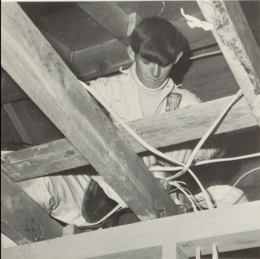
Joe Scholl splices wires in the attic in the electrical junction box.
