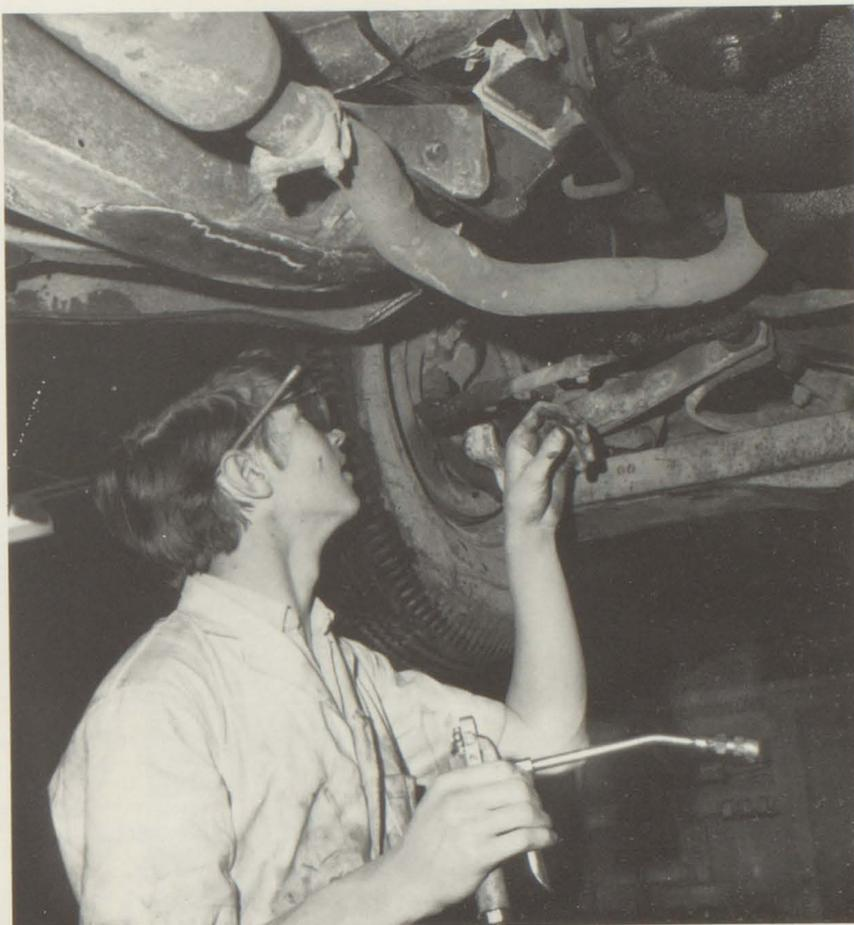
Greasing an axle is an important step in the maintenance of the car belonging to Carl Watters.
