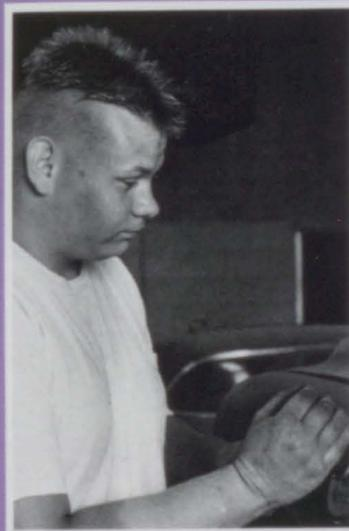
John Grit prepares a car for a new paint job by sanding the left front quarter panel.
